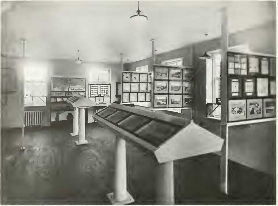
Fig. 23 The British Mosquito Control Institute demonstration museum
